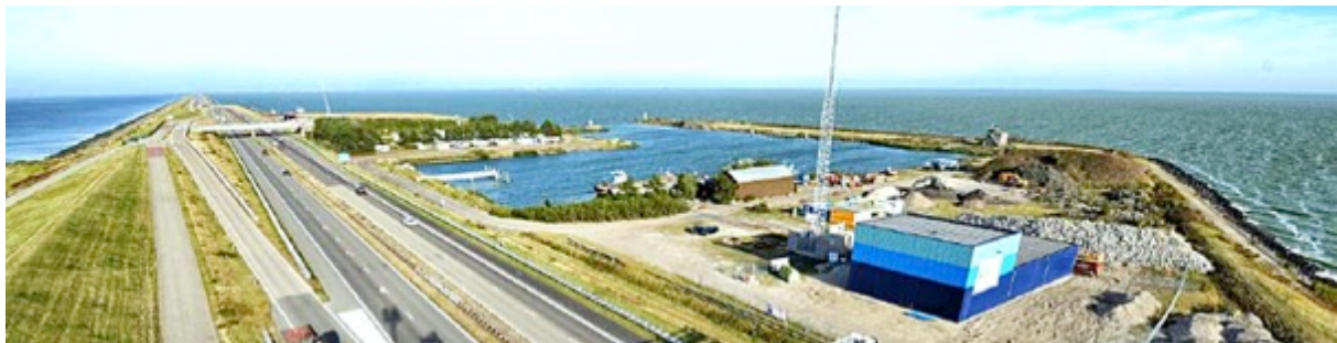
Figure 9: Pilot plant facility for reverse electrodialysis at Afsluitdijk, The Netherlands. Salt water supplied from the left side of this dam (Wadden sea), while fresh water is obtained from the right side of the dam (IJsselmeer).
